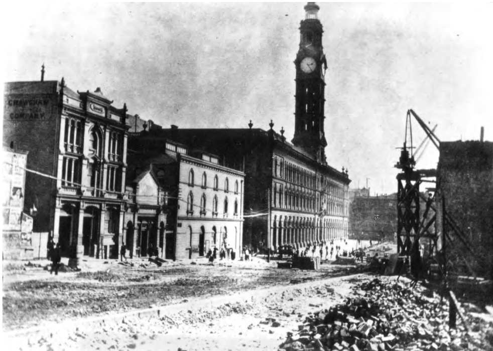
46 The widening of Moore Street in 1892. The buildings in a state of dereliction were destroyed by fire in 1890.
