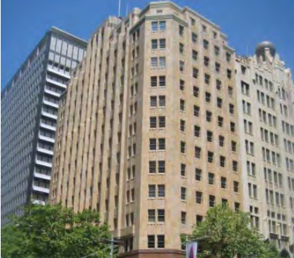
APA Building, 53-63 Martin Place
