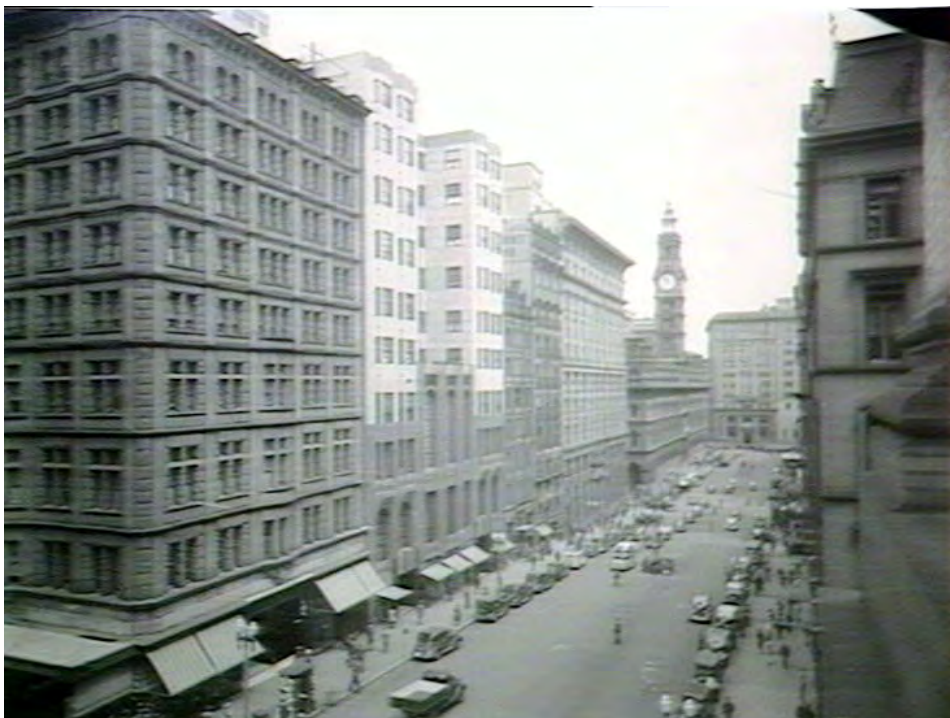
52 The former Australia Hotel at 19 Martin Place. Erected in 1932 to the design of architect Emil Sodersteen, demolished in the early 1970s for the MLC Centre. The guest rooms of the upper floors were naturally lit by the recessed light well. The street level continued the pattern set by its predecessors. Source: State Library NSW – Small Picture File – Sydney Streets – Martin Place
