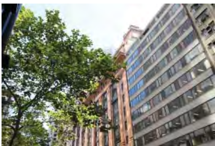
50 Martin Place - north-east lift overrun tower
